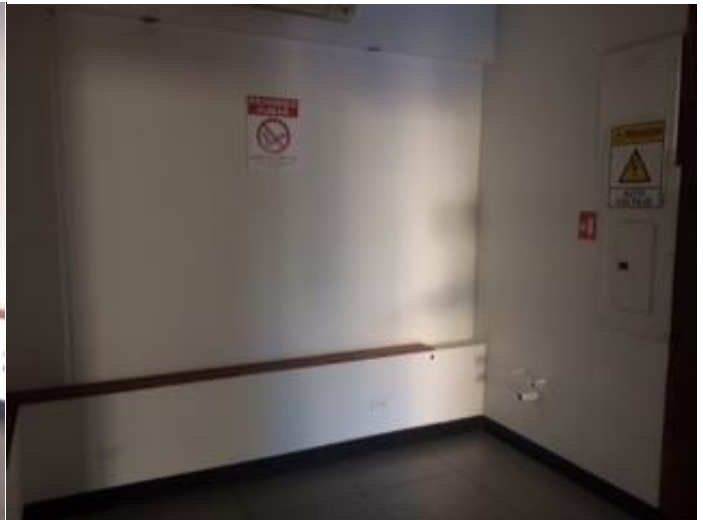
Small office looking at rear and right wall
